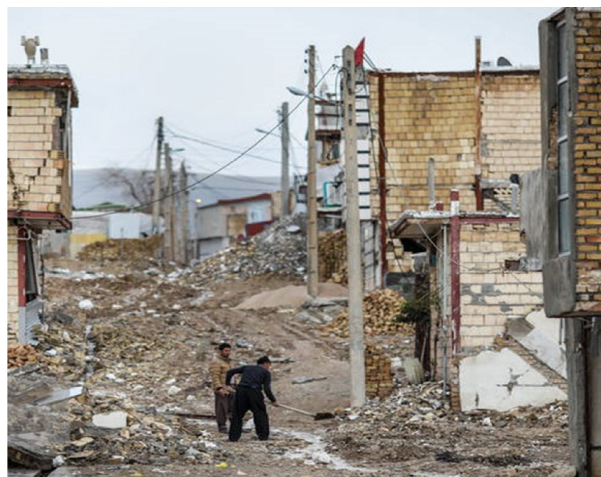
Figure 16. Access Blocked (Source: Authors)
