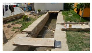
**Figure 18.** Clogging of water in canals (Source: Authors)
