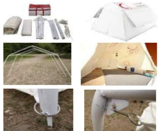
Figure 7. From the top right: exterior view, general requirements, interior view, tent frame, roof connections, and base connections in tents Type 2
