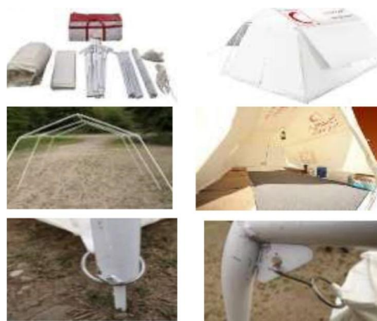
Figure 7. From the top right: exterior view, general requirements, interior view, tent frame, roof connections, and base connections in tents Type 2
